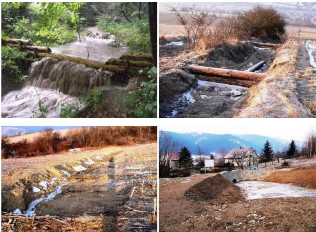
Figure 32: Water retention measures in the Kysuca river basin (Snežnica, Dunajov, Skalité, Stará Bystrica) and their functionality during intense rainfall. (Photo: Kravčík, M., Šuty, P., Petrákova, D.,)
