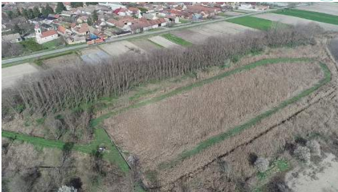
Figure 36: Constructed wetland, NBS wastewater treatment facility (photo by Atila Bezdán, Jovana Bezdán-UNSFA)
