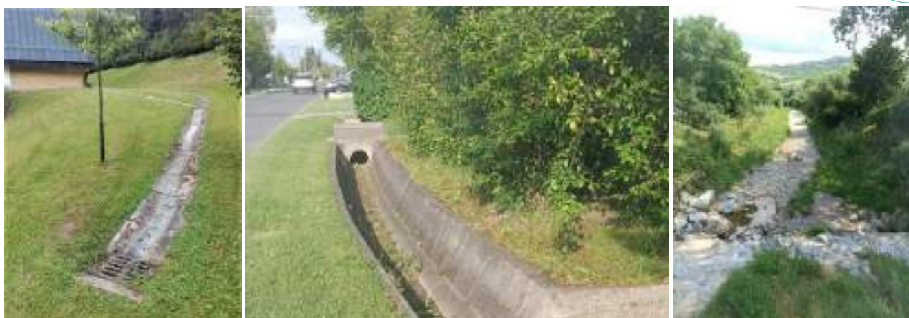
Figure 26: The principle of the old water paradigm in practice. We get rid of rainwater as something that makes our lives uncomfortable. We do not see the connection that all the water we have in Slovakia comes from rain (Photo: Kravčík., M.,)
