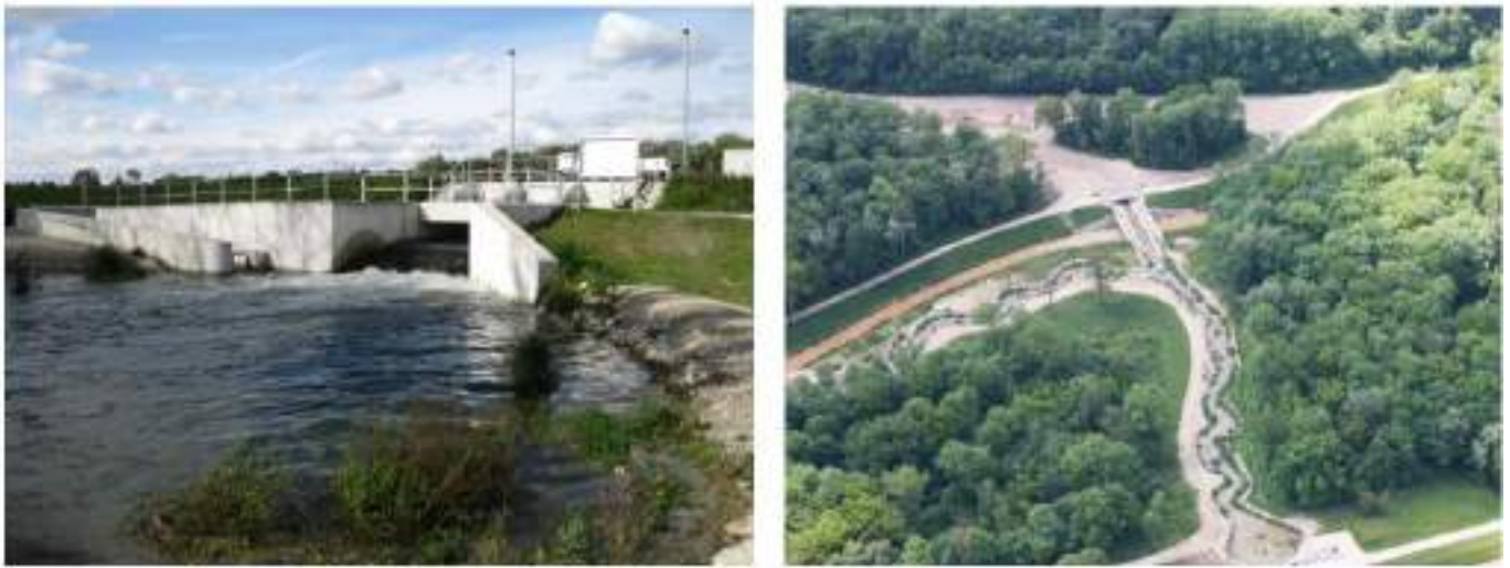
Figure 21: Left: Diversion structure with stilling basin and fishway. Right: Ottheinrichbach with short connection to the heavily turbid Längenmühlbach and trough bridge. In the background, the basin pass after the trough bridge (still without water) and the upper flood basin (area behind the detached group of trees), which is to lead the water into the floodplain forest during ecological flooding (photos: Peter Fischer).
