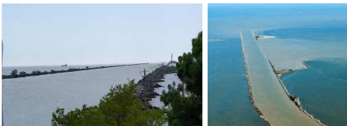
Figure 52: Sulina branch extended into the sea with stone embankments (source: a) NIHWM, 2021; b) https://dunare.ro/sulina-oras-din-romania/bara-sulina/ )
