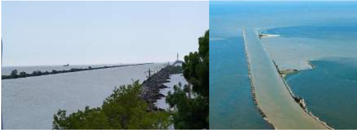
Sulina branch extended into the sea with stone embankments (source: a) NIHWM, 2021; b) https://dunare.ro/sulina-oras-din-romania/bara-sulina/ ) a) b)
